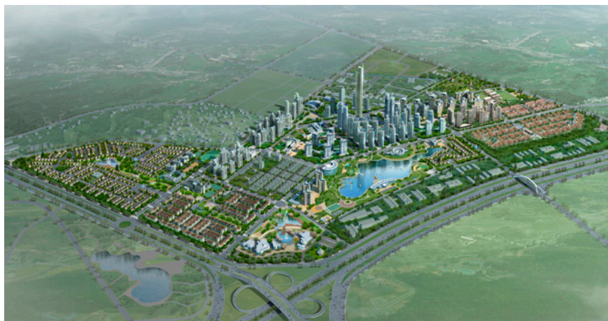
Figure 4. Perspective view of the Splendor New Town (Copyright POSCO Engineering and Construction Co.).
