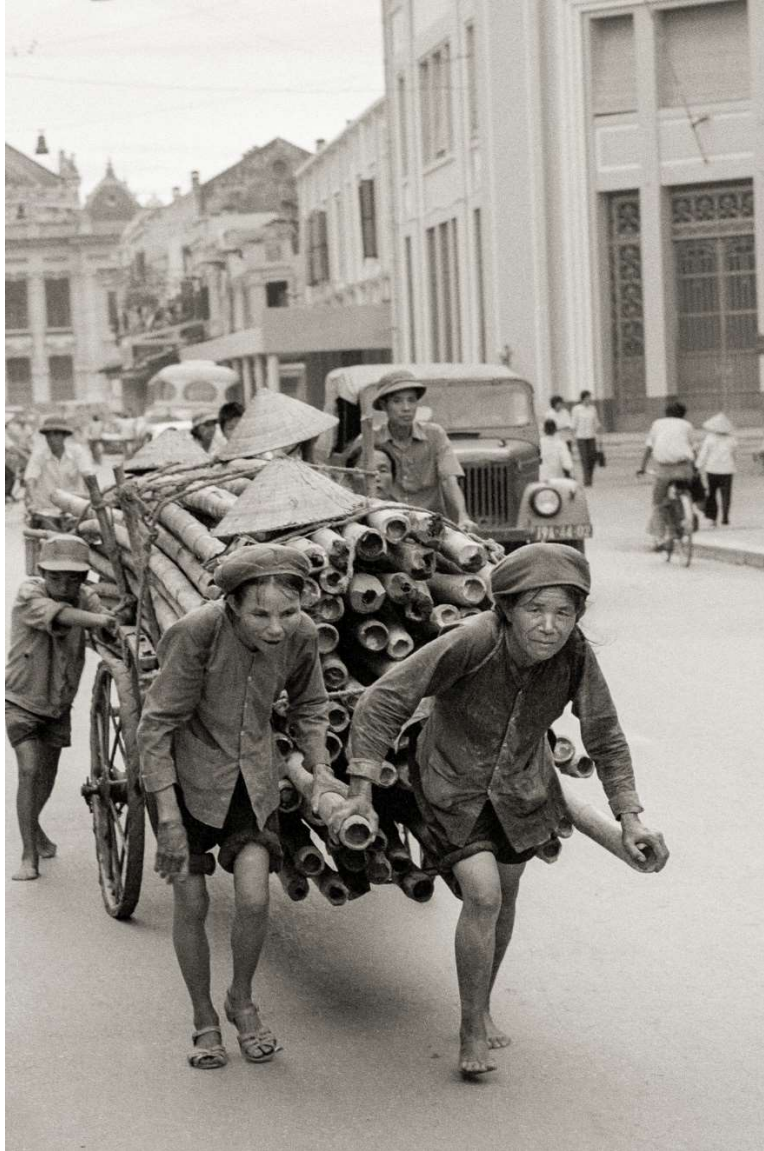
A load of bamboo. Bamboo was floated down-river for use as scaffolding on the city's many building sites. Tran Tien, then as now, was the city's smartest street, making the plight of these women all the more poignant.
